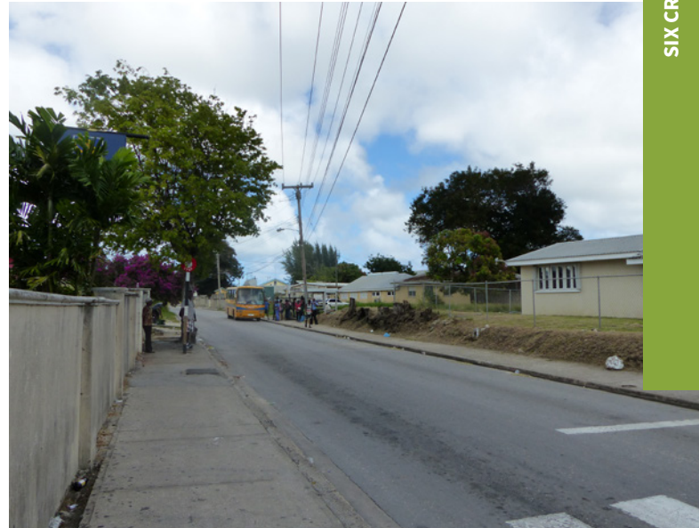
Street frontage of Civic Campus on Congo Road
