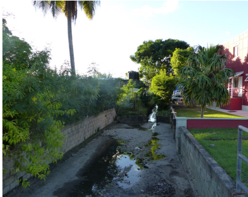
➤ Culvert leading to the outlet at the Public Centre
