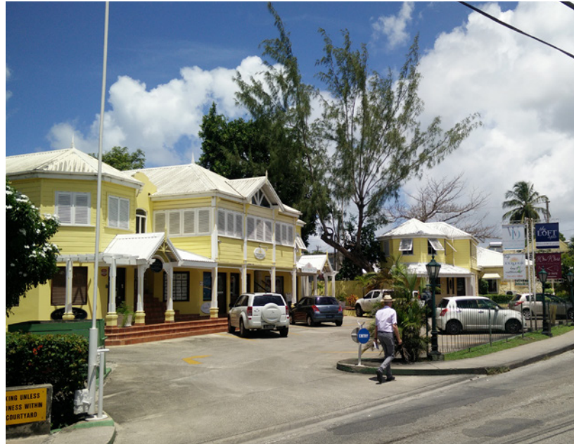
> Reused historical building, Highway 1
