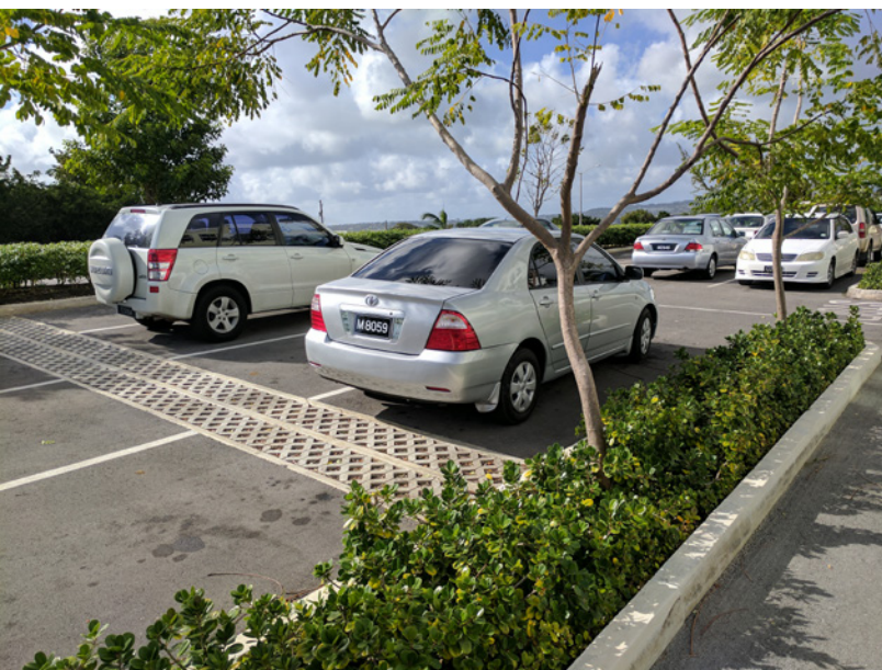
> Parking designed to address stormwater, The Pine
