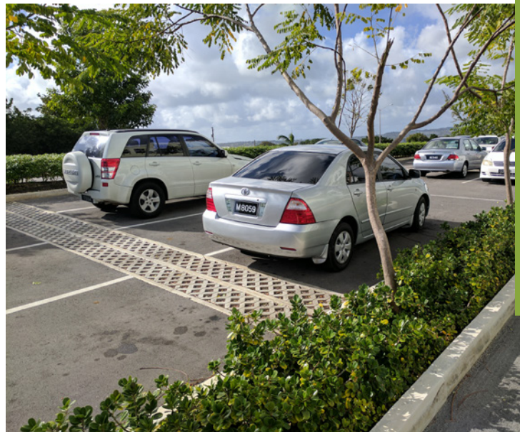
➤ Surface parking lot with porous paving and landscaping
